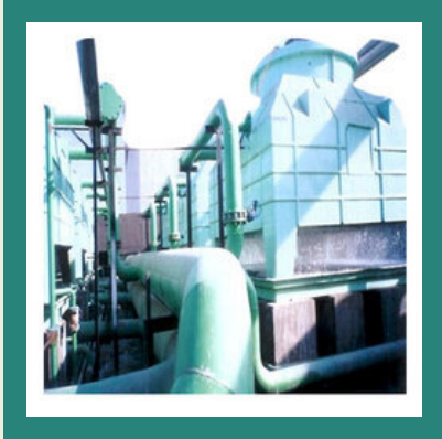
Cooling Water Treatment Chemicals
